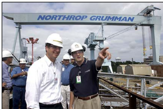
Scott Stabler, vice president for the CVN 77 Program (in blue shirt), showed Sen. Allen around the north yard, where the George H. W. Bush is under construction.
